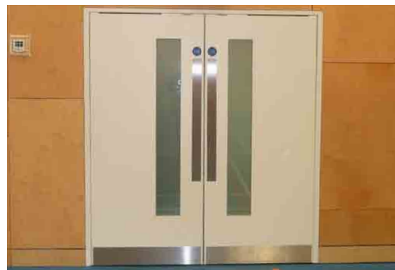
Standard proprietary flush door with a flush viewing panel, opening outwards away from the sports hall
