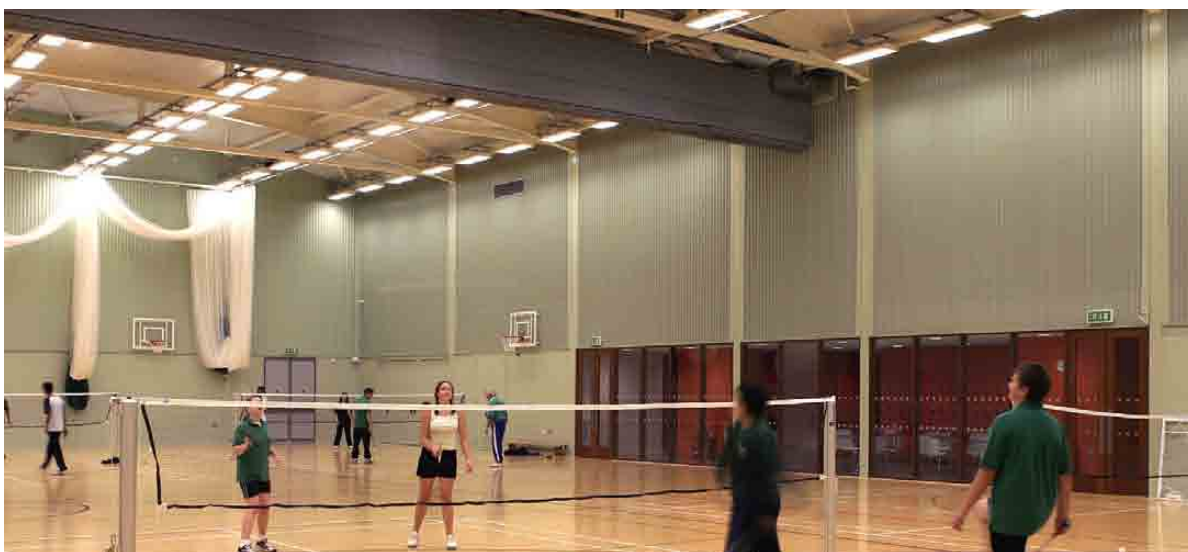
Acoustic dividing screen at the centre point of a 6-court hall on a school site allows the space to be divided into two teaching spaces
