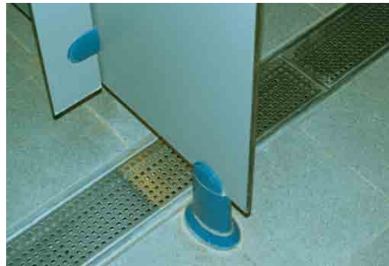
Floor channels with bucket gullies and lift-off grilles give effective drainage in shower and other wet areas. They require regular cleaning
