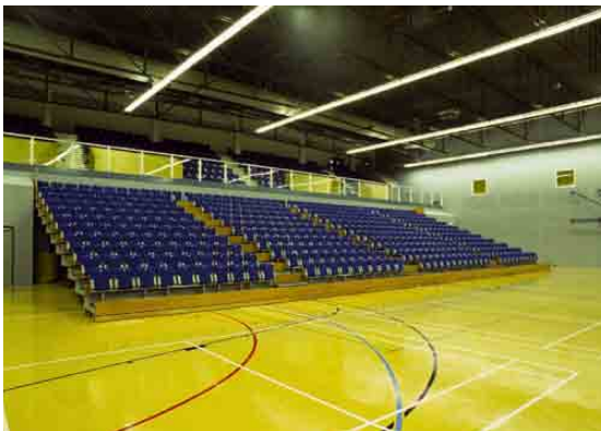
Bleacher seating integrated into the side wall and access gallery above
