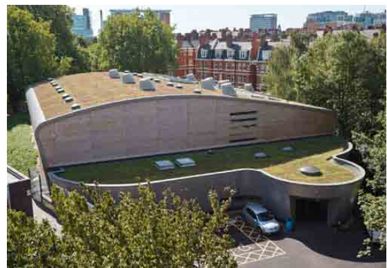
Natural ventilation towers in roof to give controlled ventilation and compensate for the heat loads from occupants, artificial lighting and solar gain, and anti-glare roof-lights to supplement the artificial lighting
